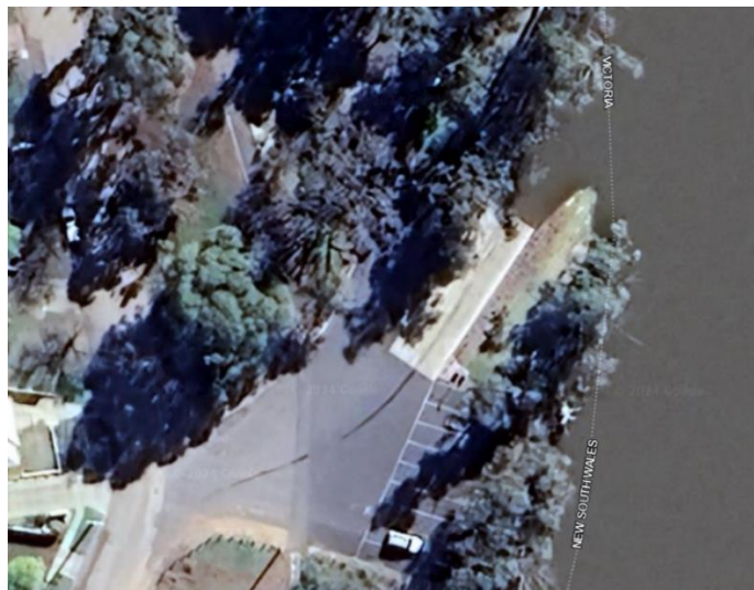
Figure 3 – Existing Boat Ramp & Parking Facilities, Milloo Street Boat Ramp (Source: Google Earth, as accessed 25/07/2024)
