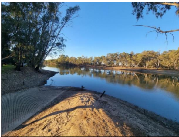
Figure 4 – Toe of Existing Boat Ramp Looking downstream (northerly)
